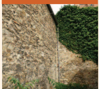
Fig. 52 Limestone tenement and outbuilding walls located west of St Aldates.
