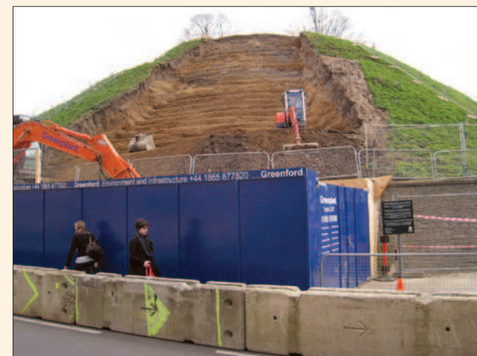
Fig. 17 Repair works to the Norman motte in 2008.
